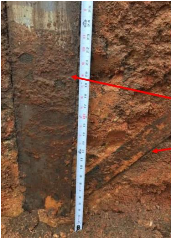
Figure I-15 Structure 2-192: Uniform Below Grade Corrosion
