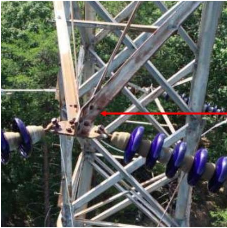
Figure I-14 Structure 2-175: Rust at Joints and on Steel Members
