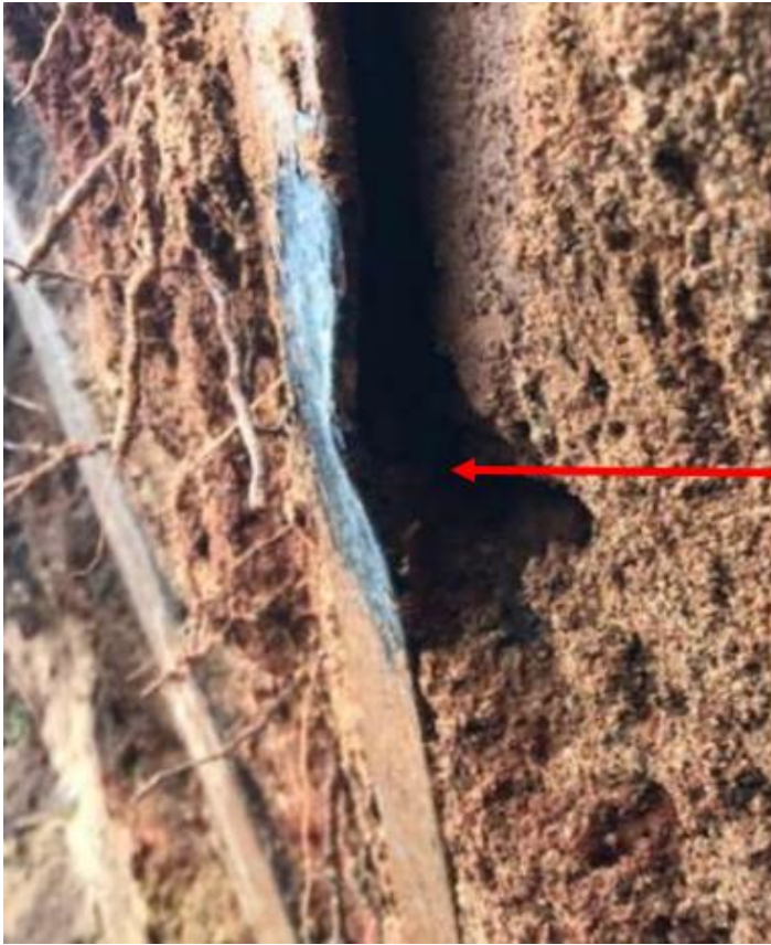
Figure I-16 Structure 2-193: Deformation of Below Grade Steel Member
