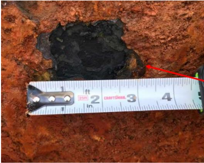
Figure I-9 Structure 2-60: Below Grade Pitting
